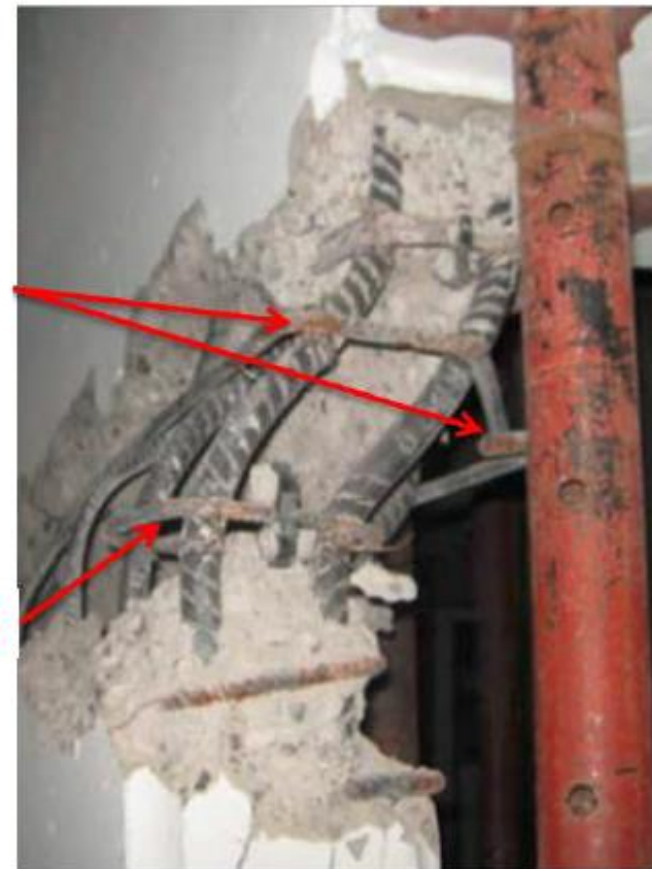
Figure A-11 Undisclosed Building A (Building No. 5) – wall reinforcing details and observed damage at the wall boundary (photo courtesy of Carl Luders).
